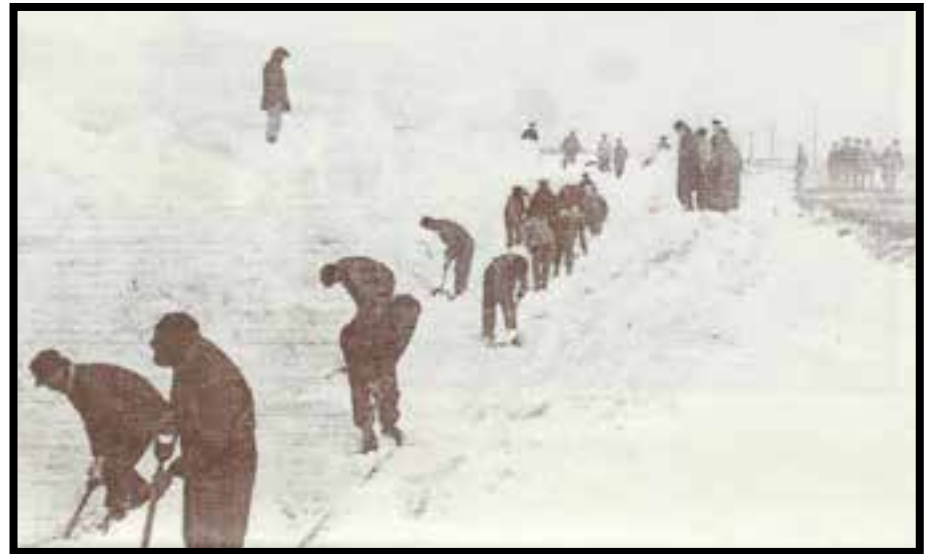
Clearing the train track. Photo courtesy of Merlin Platte
